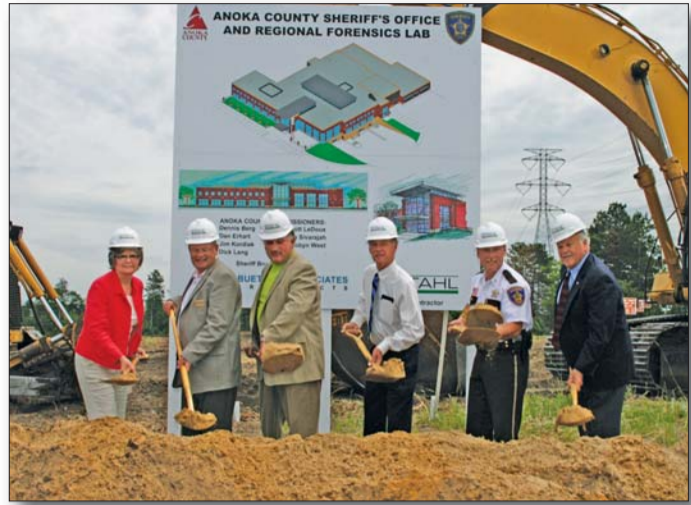
Attending the ground-breaking ceremony for the new public safety center are, from left: Anoka County Commissioners Robyn West, Dennis Berg, Scott LeDoux, and Jim Kordiak; Anoka County Sheriff Bruce Andersohn; and Anoka County Commissioner Dan Erhart.
